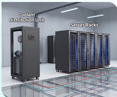
Coolant Distribution Unit
