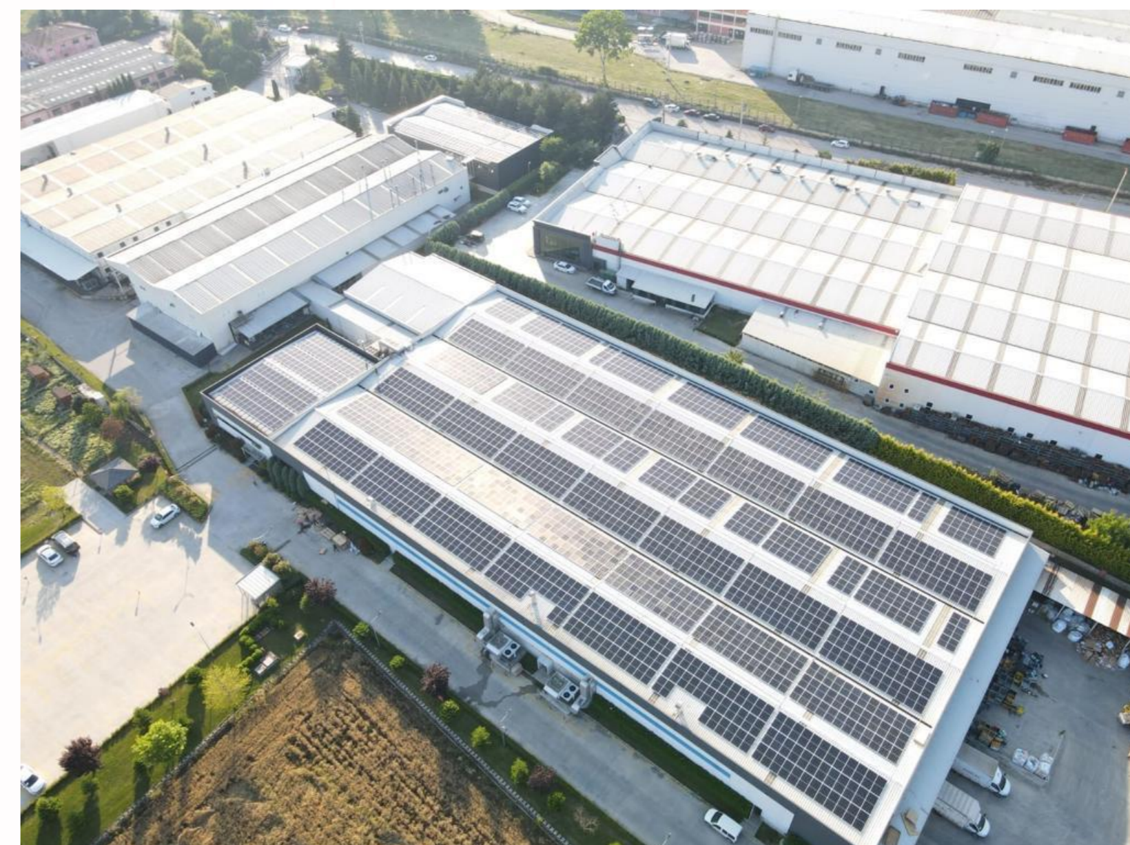
Alpplas Bolu Plant
